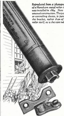
Reproduced from a photograph of a Hartshorn metal roller that was installed in 1864. Note the unusual construction. The pawl, or controlling device, is part of the bracket, rather than of the roller itself, as is the case today.
